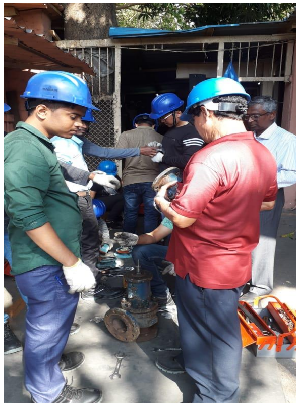
Students performing maintenance of valves
